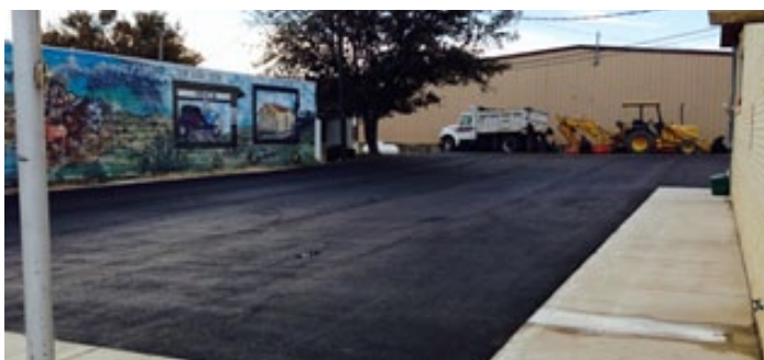
The new parking lot next to the ED building is sponsored by both the EDC, CDC and Parks Department. The parking lot has made a huge difference to the downtown area! Concrete work has been started at the Old Fields for new backstops and dugouts!
